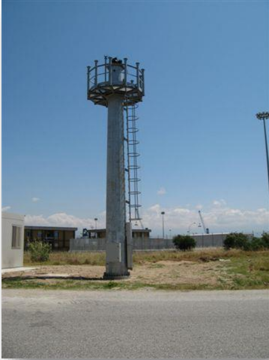
Figure 6: Off airfield security tower mount.
